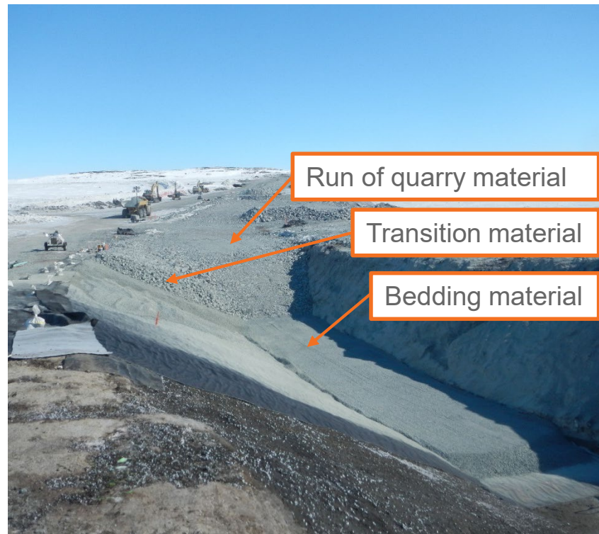
Backfilling of key trench above liner
