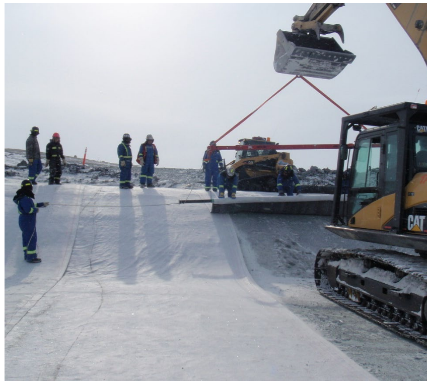
Liner installation in key trench
