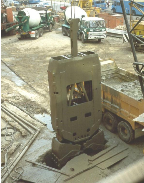
CLAMSHEL BUCKET SLURRY WALL (Urban Area)
