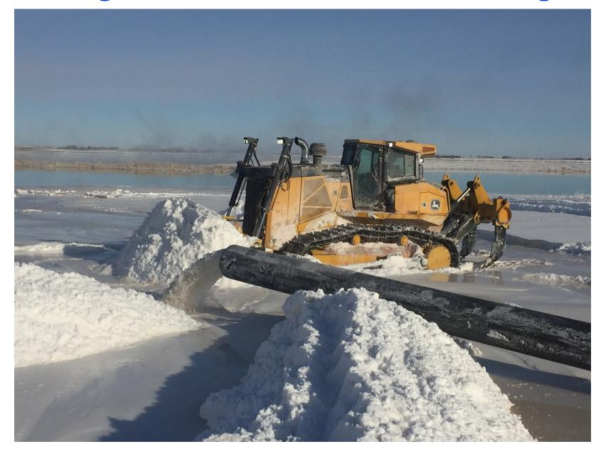
Moving tailings to build elevated platform for discharge line
