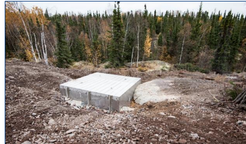
Completed cap at Ace 130 Raise
