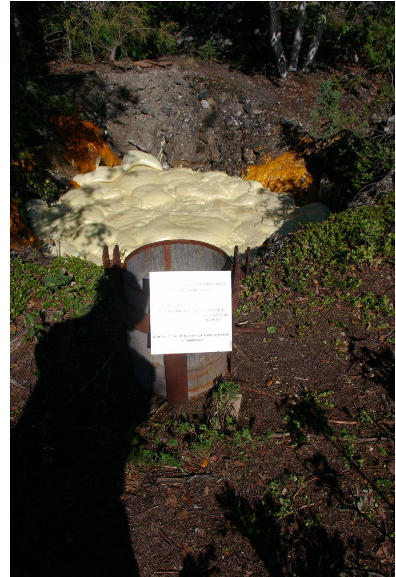
Expandable foam in northern Saskatchewan (Non-Beaverlodge) used as a temporary closure method to address immediate safety risk photo by Michael Webster
