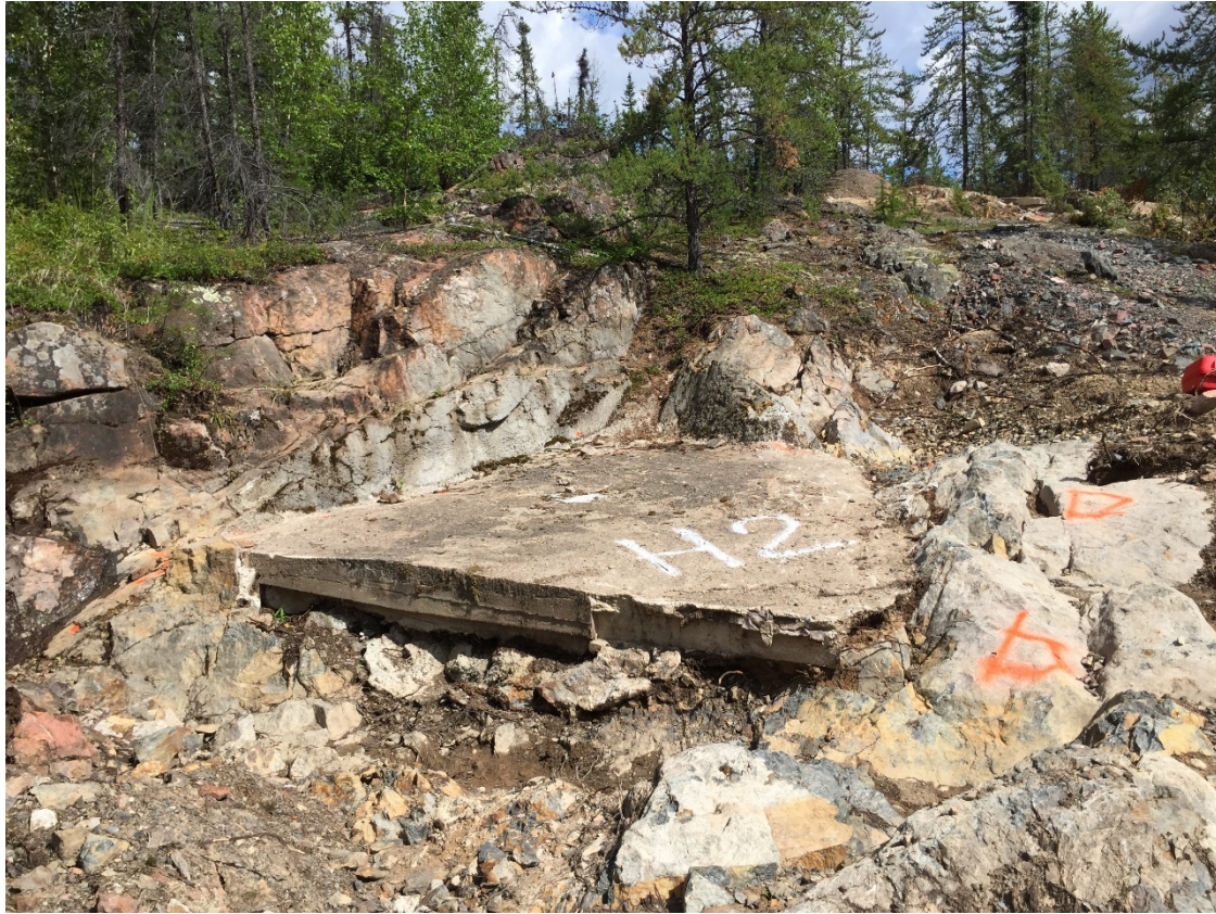
Cap cleaned off with bedrock expose
