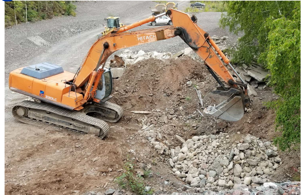
Boulders placed around key boulder
