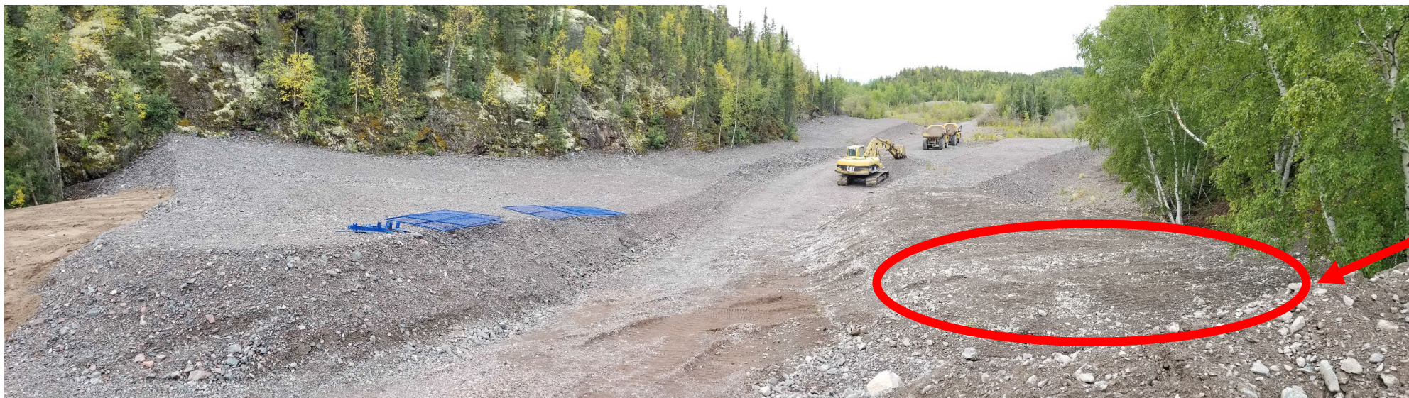
Location of Ventilation Raise graded to surrounding area
