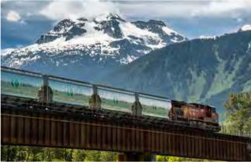
Reliable rail infrastructure is essential for moving potash to market. Photo courtesy of Canpotex.
